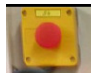
Cooling water switch-off
